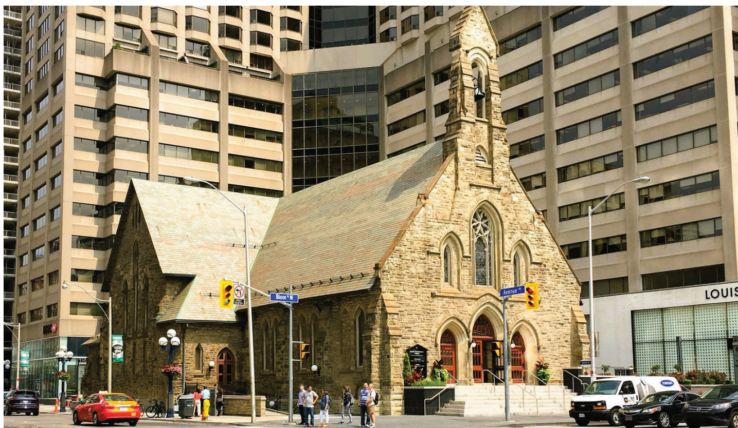
Figure 2: Episcopal church of the Redeemer, Toronto –a place of worship marooned in a high-density urban environment (source: Robin Stevens, 2017)
